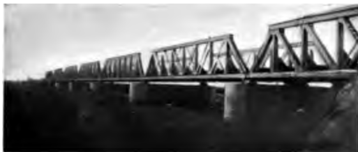
THE YANGTSUN RAILWAY BRIDGE.
