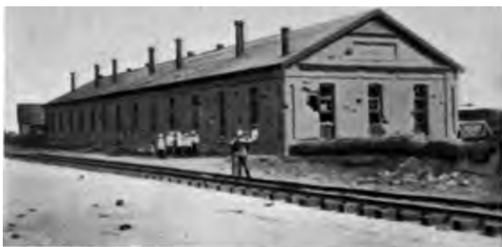
HEIXIN RAILWAY STATION SHELLED
