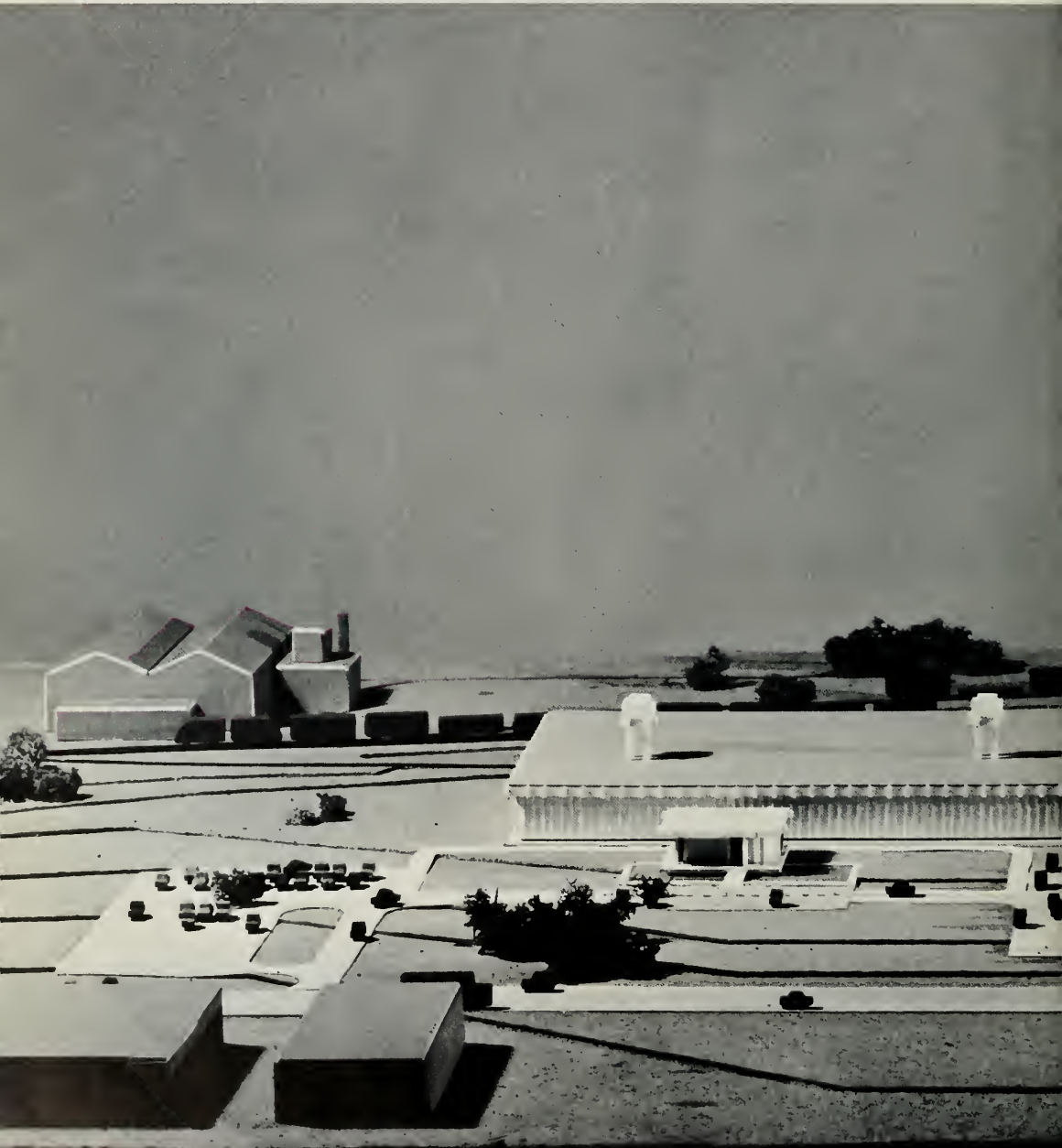
over-all view of site looking toward front entrance
