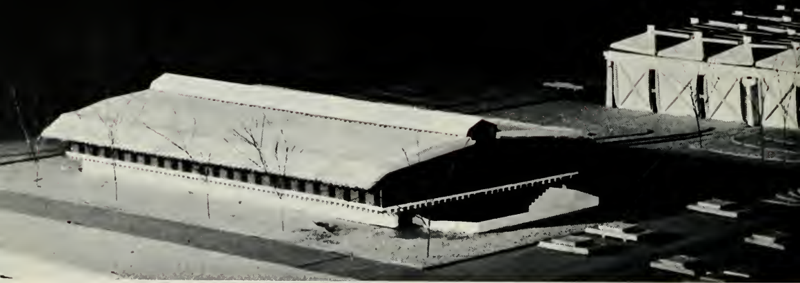
overall view of plant from above
