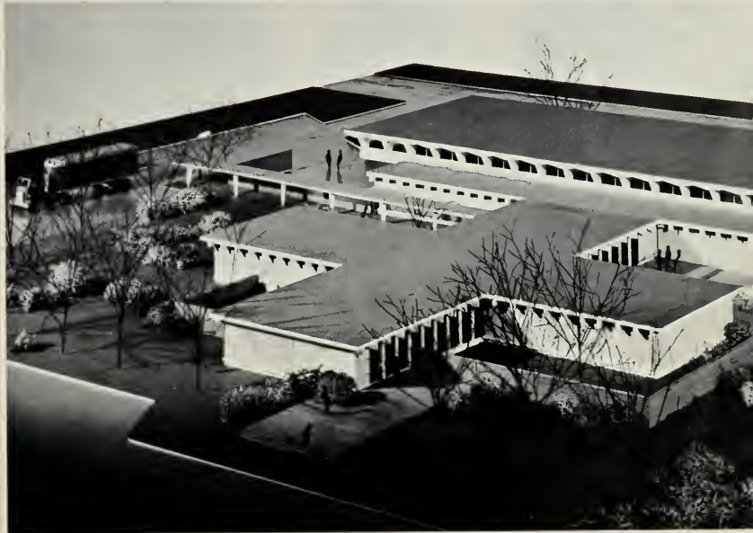
VIEW FROM ENTRANCE (ABOVE)
