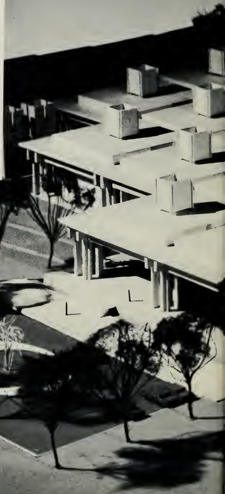
Model of two typical bays showing elevation (lower) and structure with roof removed (upper).
