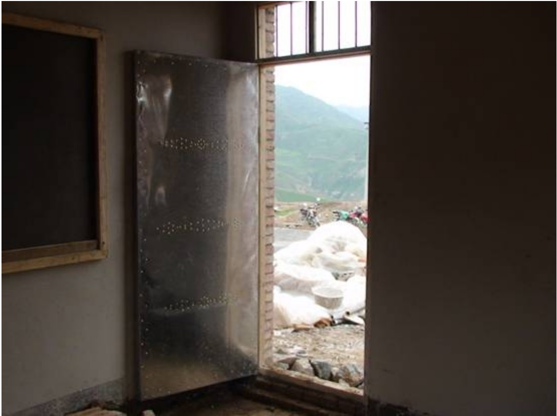
Wood doors covered with metal.
