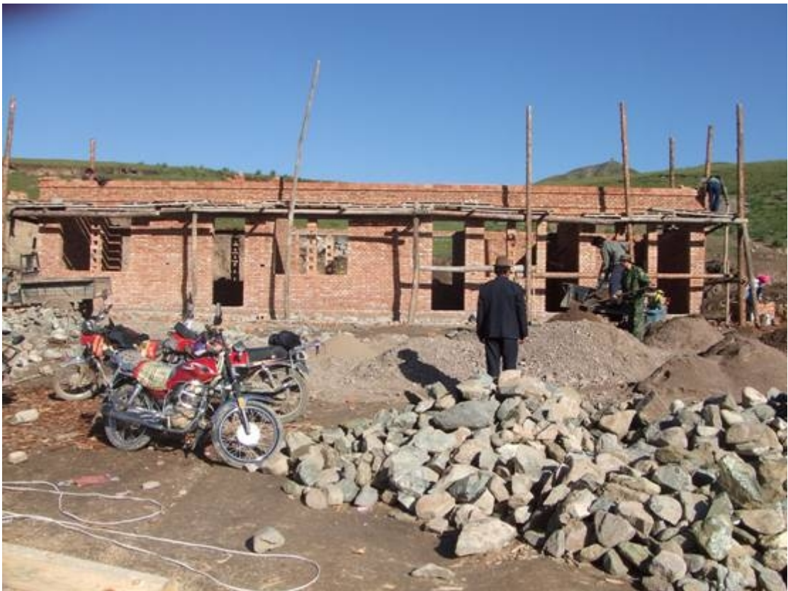
The construction group builds brick-walls.
