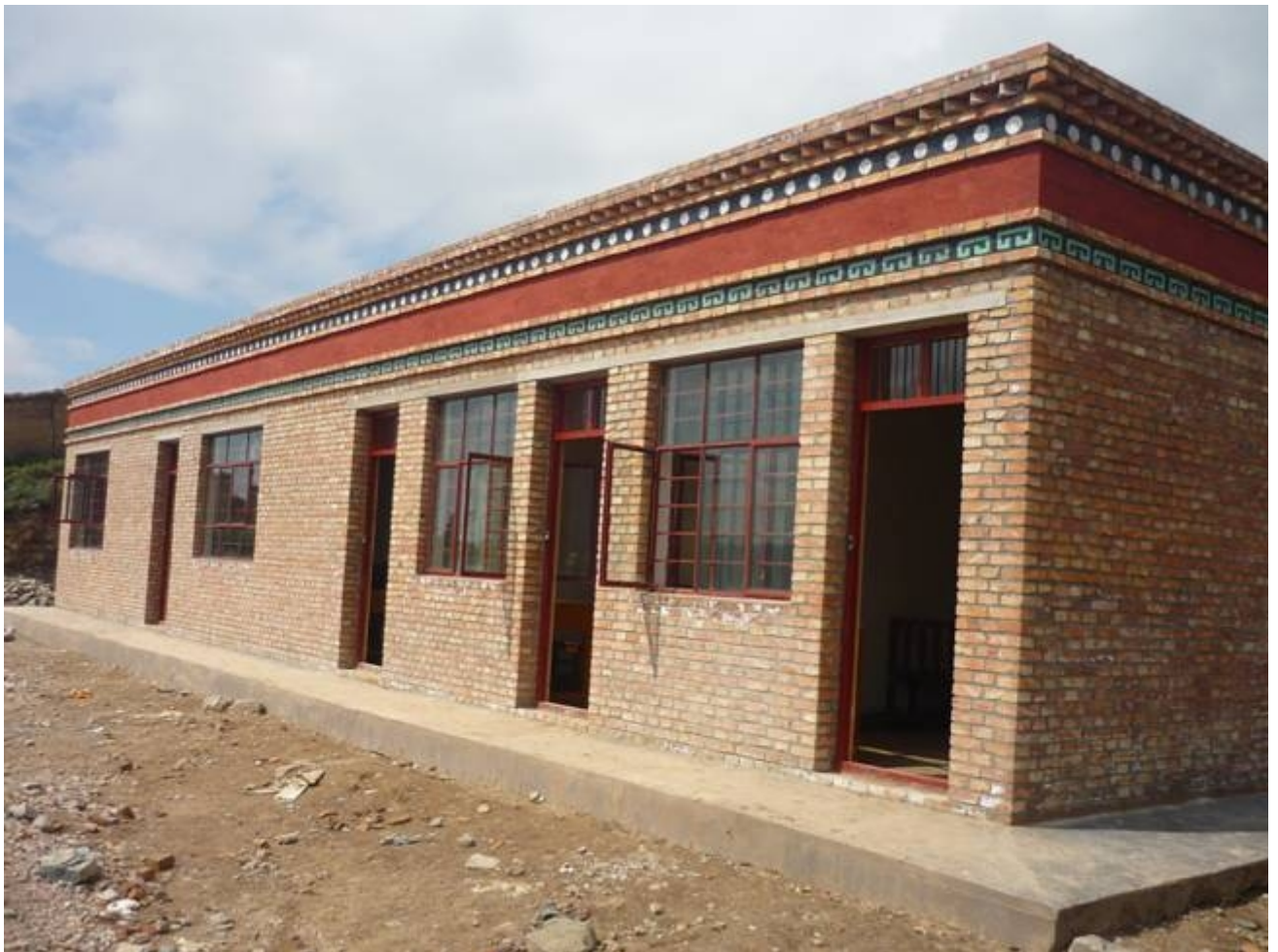
Front view of the new school building.
