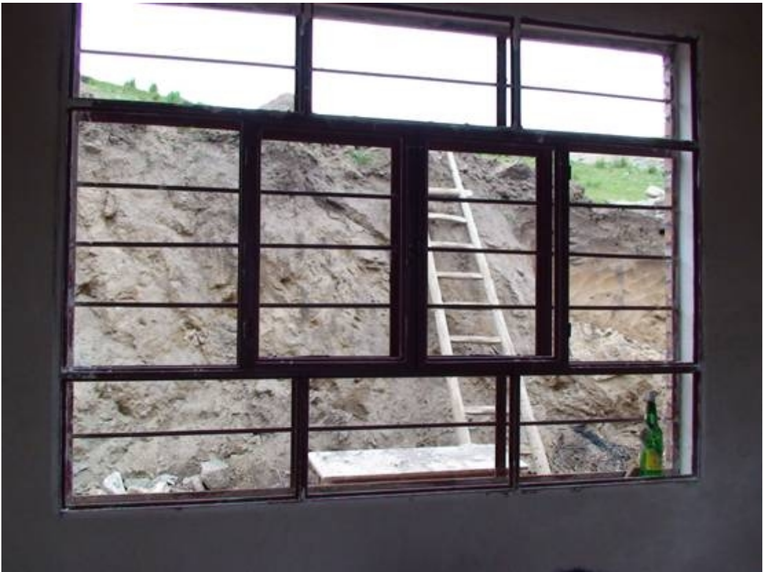
Metal window frames after installation.
