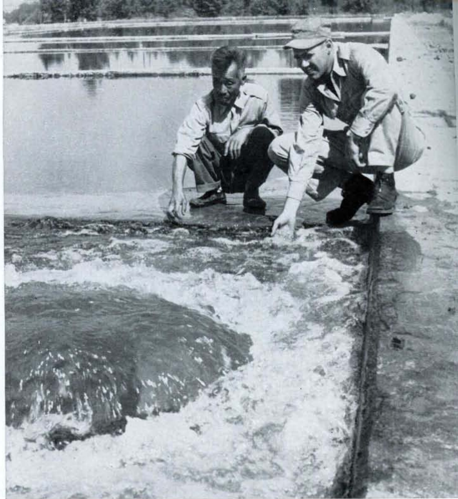
DURING THE WAR, 39 WATERWORKS WERE BADLY DAMAGED. BY MARCH 1954, U. S. HAD REBUILT AL
