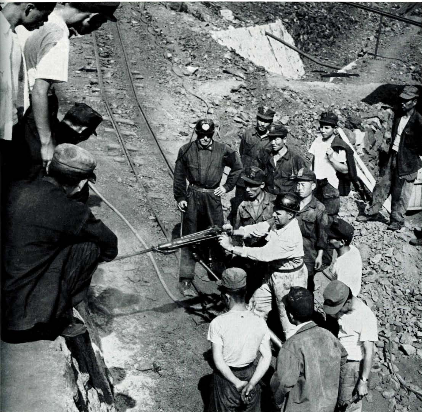
AN UNKRA COAL MINING CONSULTANT DEMONSTRATES THE OPERATION OF A MODERN JACKHAMMER TO A GROUP OF KOREAN MINERS AT EUNSONG.
