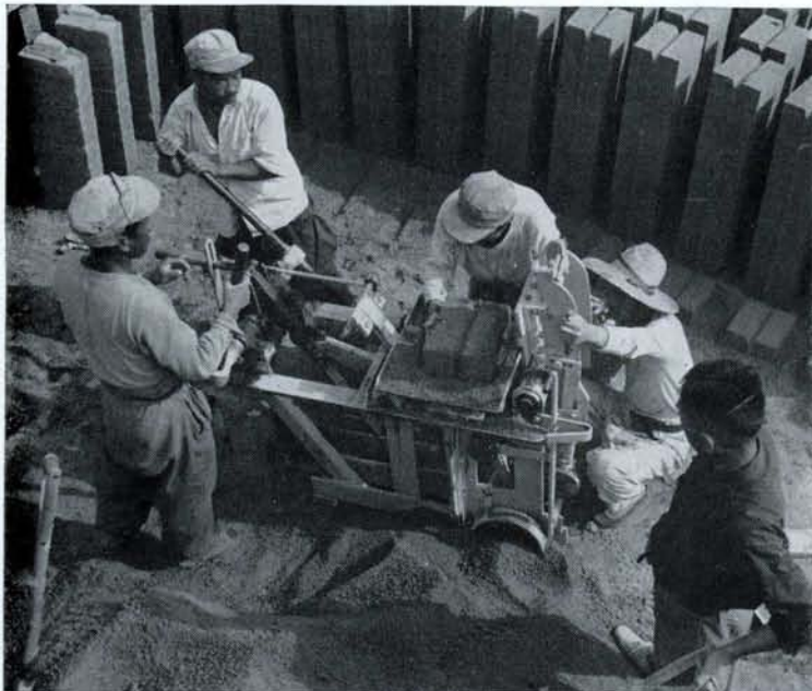
KOREAN WORKERS OPERATE ONE OF 100 UNKRA EARTHBLOCKING MACHINES.
