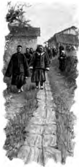
A Road Paved with Stone Slabs Showing the Groove Cut by Wheelbarrows
