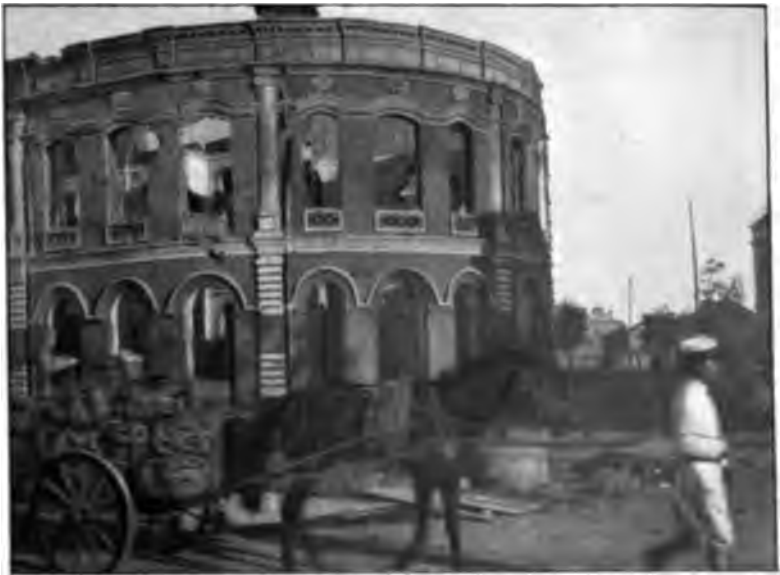
RAILWAY ADMINISTRATION BUILDING, INDOCHINA, SHOWING EFFECTS OF WAR.
