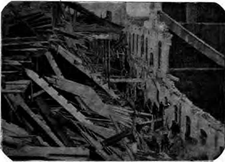
INTERIOR OF MILL AT OSAKA AFTER THE EARTHQUAKE.
