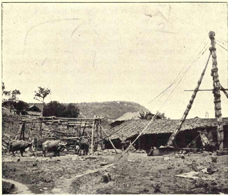
BORING FOR SALT AT TZELIUTSING.
