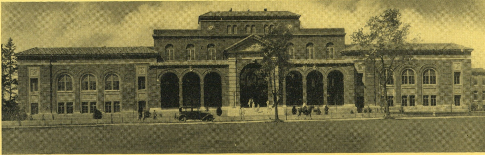
The Women's Building, architecturally beautiful and admirably adapted, through its modern facilities, organization and equipment, for the development of the health and recreational life of the women students.
