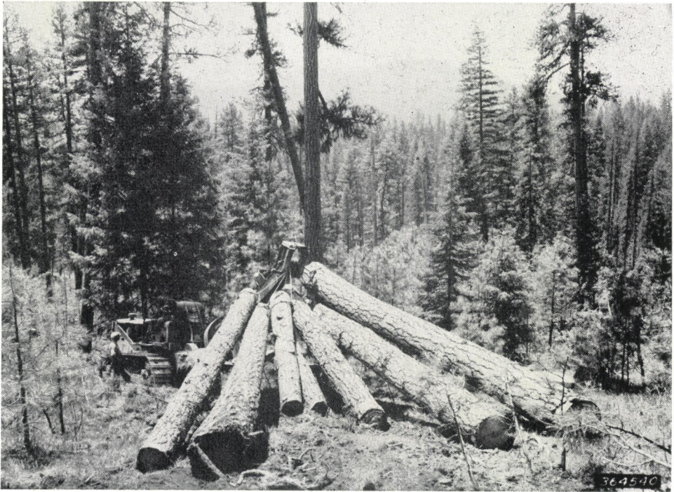
The modern "cat" logging methods are largely responsible for high daily production of logs in the forests. Here is shown in the pine country a cat tractor with arch and winch capable of hauling six or seven large logs.
