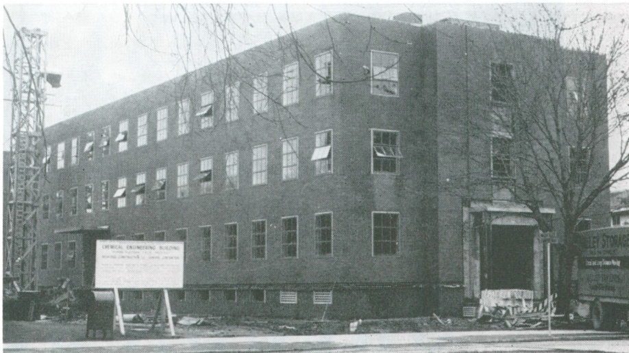
OSC's chemical engineering building should be completed sometime during the summer. Building is located between the chemistry building and library and is adjacent to the commerce building.
