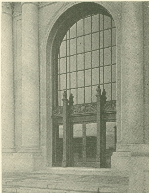
Massive columns guard the main entrance with its bronze Kalamein doors presented by the class of 1926. Note the guardian beavers.
