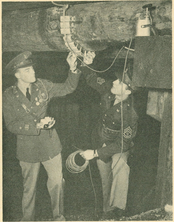
Two advanced ROTC men prepare a bridge for demolition during training for commissions in the Engineers.
