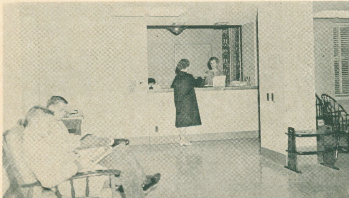
Addition to the health service building brought about spacious new reception room for students.
