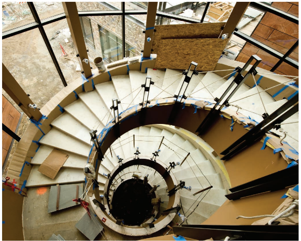
▲ Blue stone treads and a brass handrail will complete The Allison's grand spiral staircase. PHOTO BY DENNIS WOLVERTON
