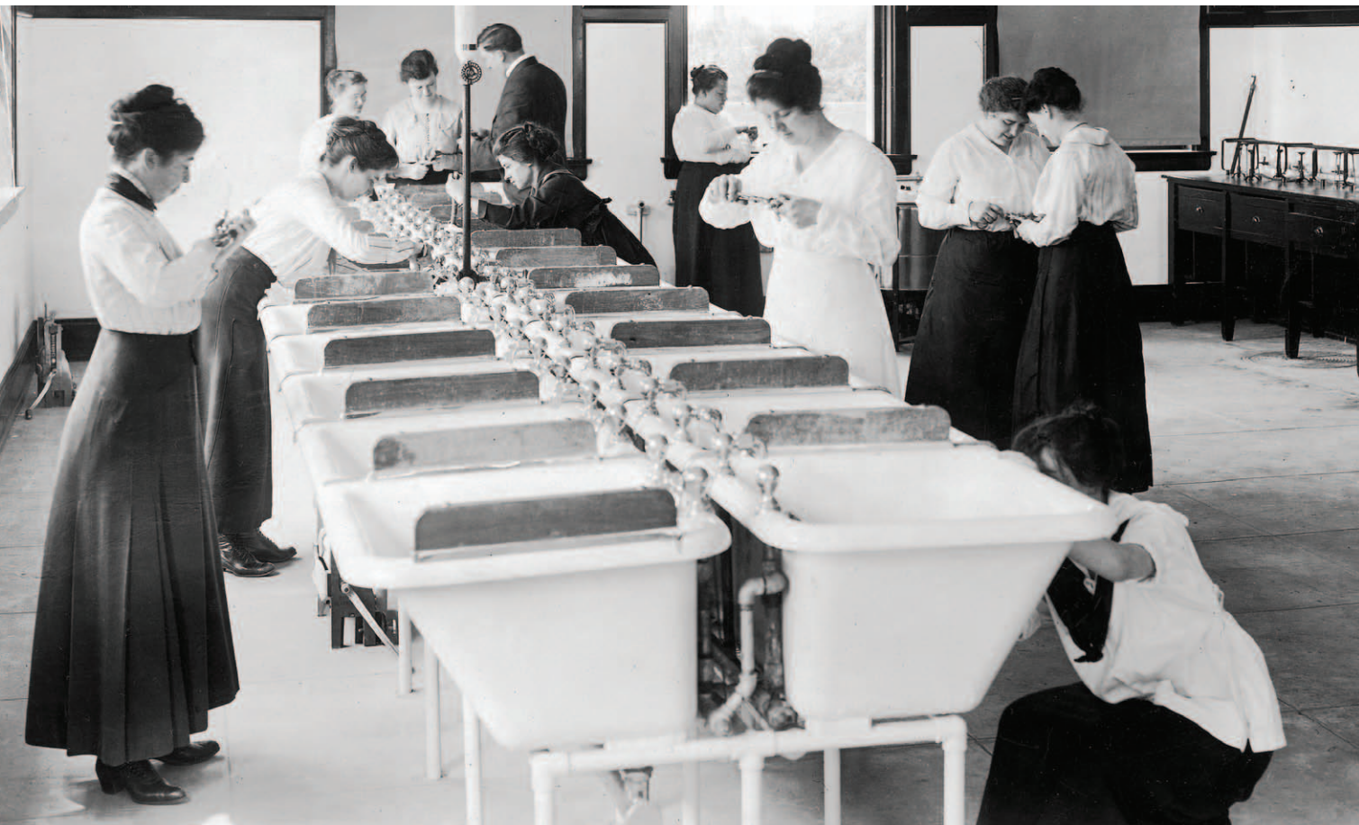
Oregon Agricultural College home economics students learn to repair faucets in a house sanitation course circa 1910, in what was then called the "Laundry Laboratory" in the Home Economics Building (now Milam Hall). PHOTO COURTESY OSU ARCHIVES HC848
