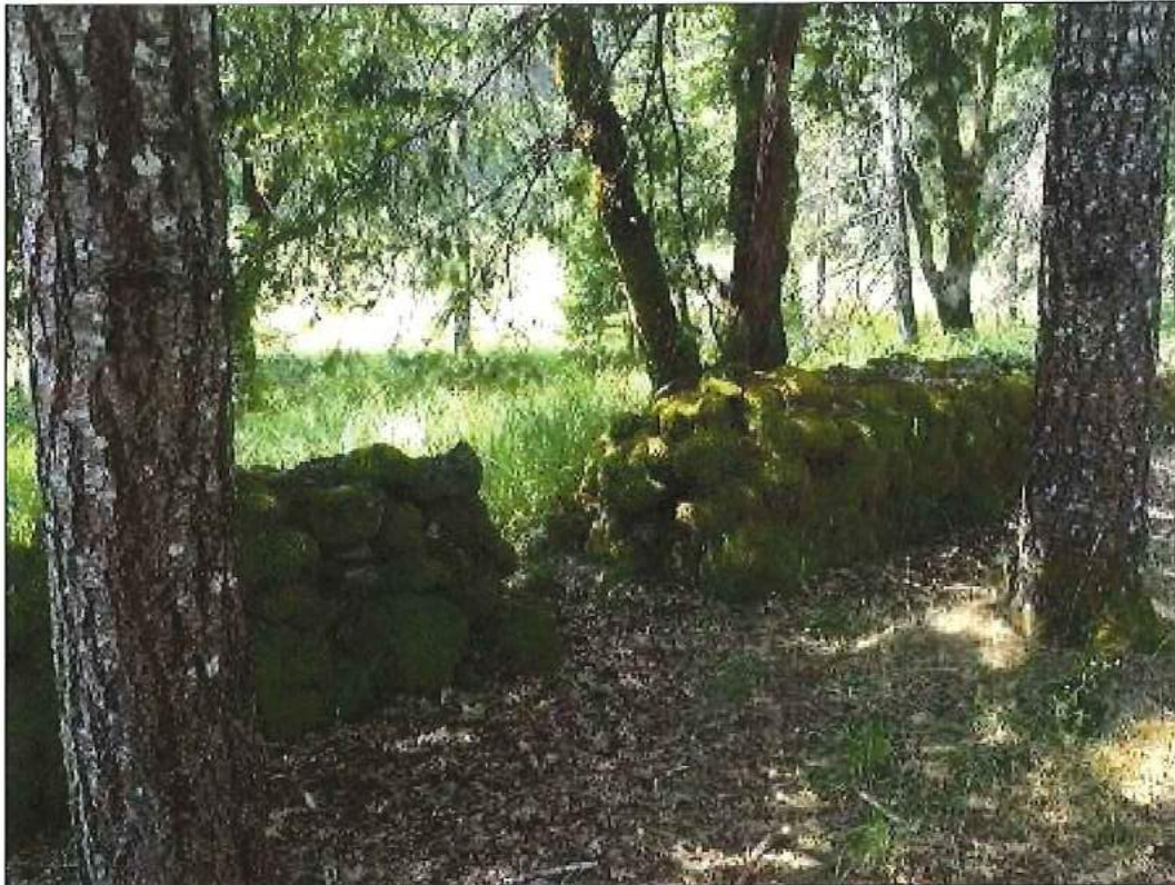
Photo 9 of 9: Dry-stack wall, camera facing west (2012).
