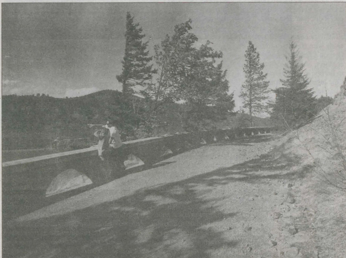
Hikers enjoy the view from Ruthton Point on an abandoned section of the historic highway just west of Hood River. Work here in the last few years has restored sections of rubble parapet wall and the Ruthton Point viaduct, which can be seen from I-84 westbound.
