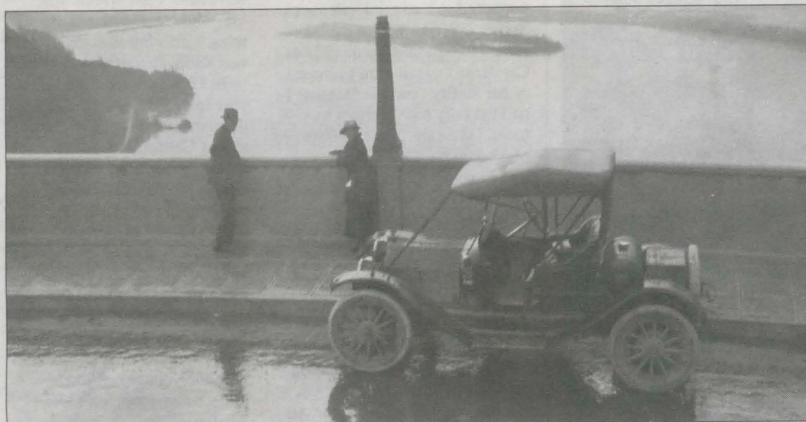
A Benjamin A. Gifford photo showing travelers along the Columbia River Highway enjoying the scenery atop Sam Lancaster's viaduct at Crown Point. OSU Archives #100
