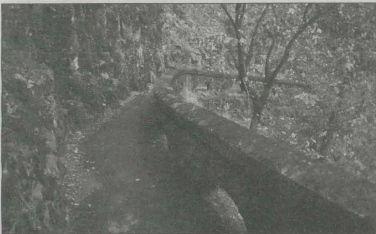
An original rubble parapet wall lines the walk down to Shepperd's Dell Falls, below the bridge of the same name.
