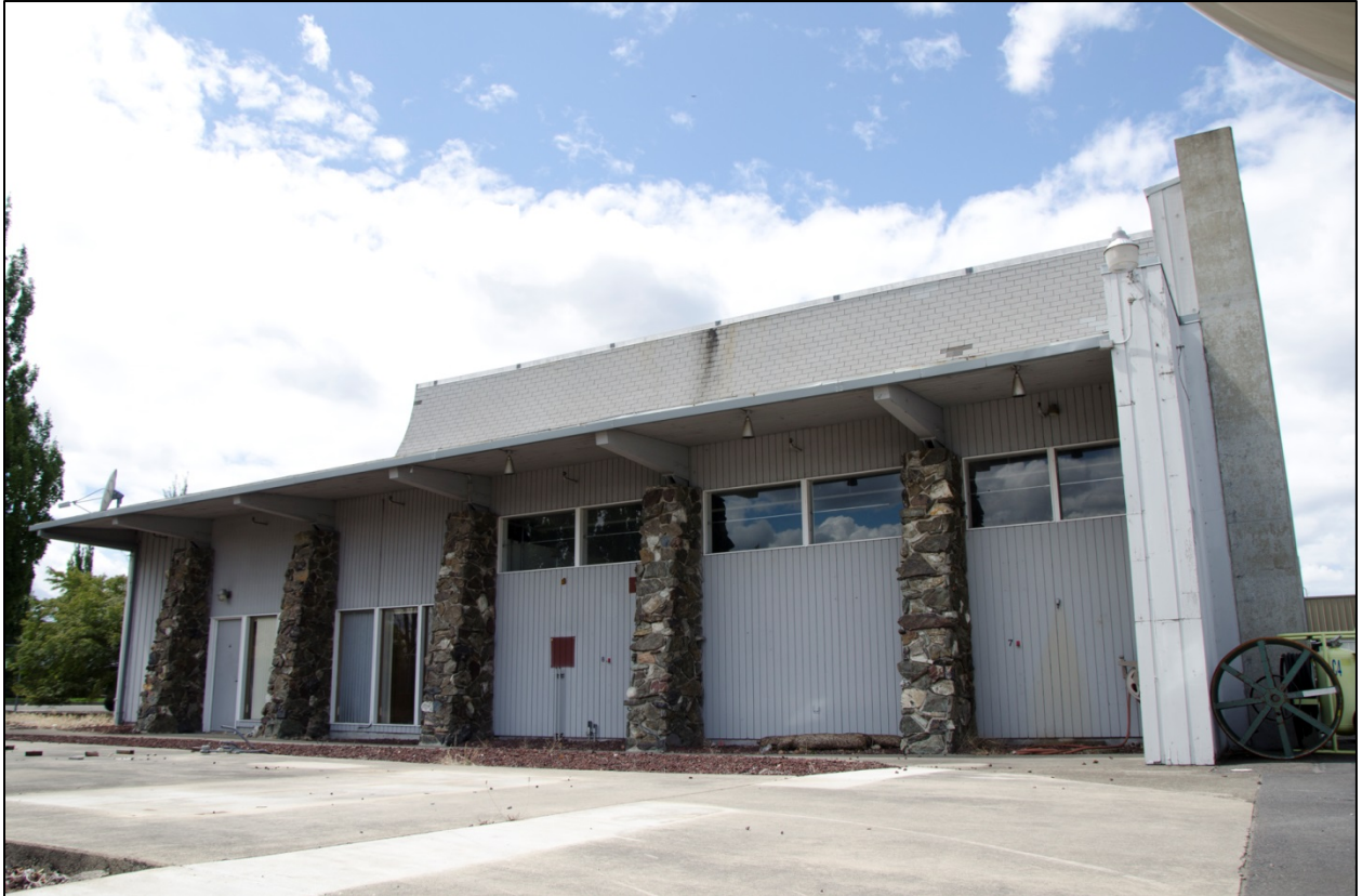
Photo 5 OR_MultnomahCounty_PortofPortlandHangar8005_0005 Hangar 8005, view to the west.
