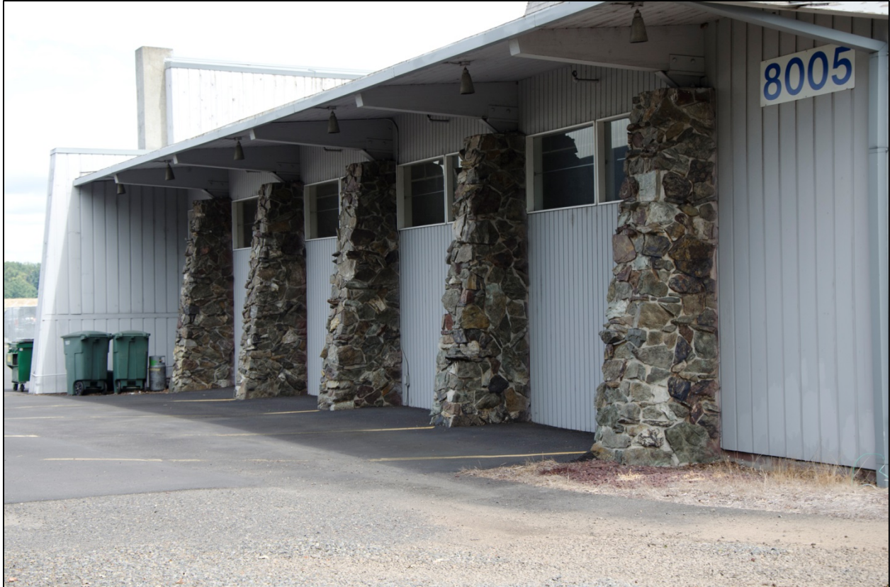
Photo 2 OR_MultnomahCounty_PortofPortlandHangar8005_0002 Hangar 8005, view to the east.
