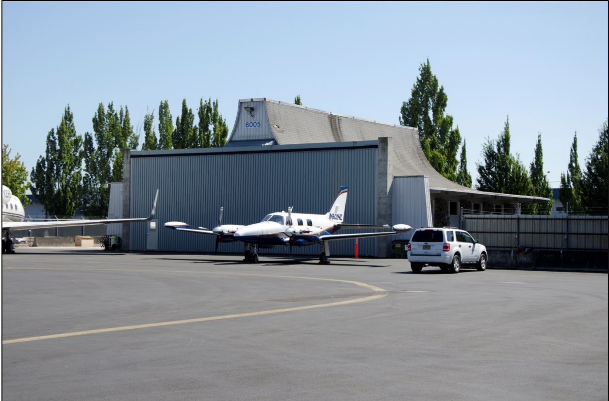
Photo 8 OR_MultnomahCounty_PortofPortlandHangar8005_0008 Hangar 8005, view to the south.
