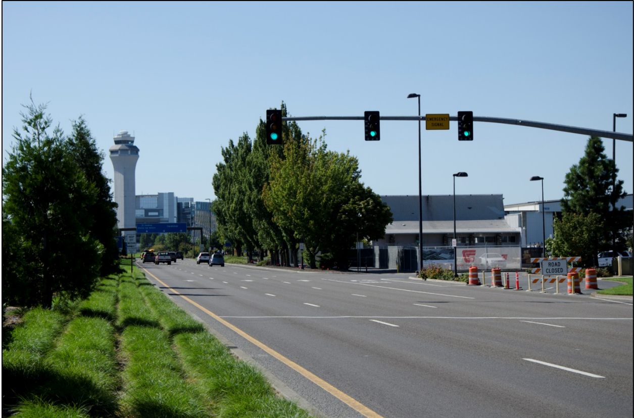
Photo 10 OR_MultnomahCounty_PortofPortlandHangar8005_0010 Hangar 8005 (right), view to the northwest toward passenger terminal and control tower.
