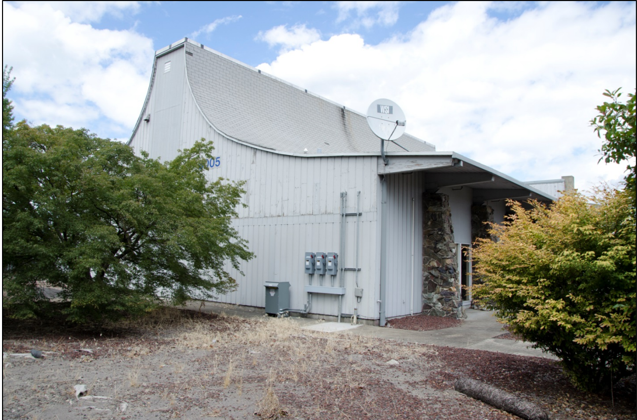
Photo 4 OR_MultnomahCounty_PortofPortlandHangar8005_0004 Hangar 8005, view to the north-northwest.
