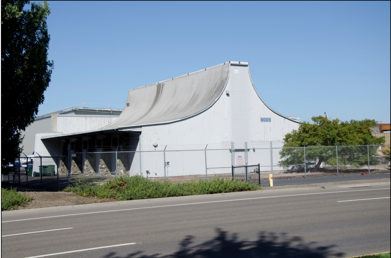
Photo 3 OR_MultnomahCounty_PortofPortlandHangar8005_0003 Hangar 8005 from NE Airport Way, view to the east-northeast.
