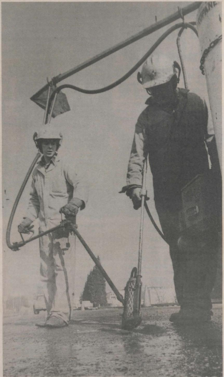
Highway road workers experiment with a new "hot lance" technique to repair road surface cracks even in cold or rainy weather
