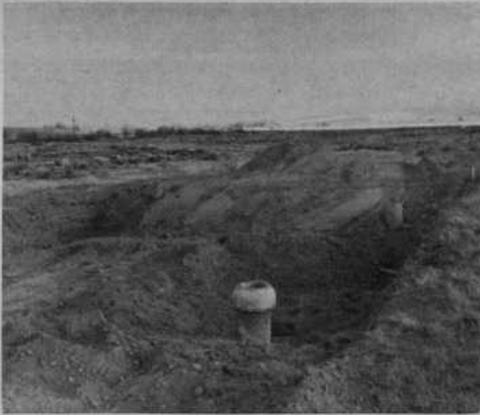
CONCRETE pipes were set in soil to allow addition of water. In dry soil 5,000 to 8,000 gallons of water were required for a 30 by 60 foot bee bed.
