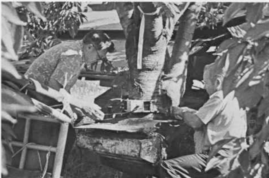
After setting accelerometers on the tree trunks (above) researchers used electronic equipment to monitor the tree movement (left). Force required to pull cherries from stems also was recorded (below).
