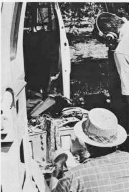
After setting accelerometers on the tree trunks (above) researchers used electronic equipment to monitor the tree movement (left). Force required to pull cherries from stems also was recorded (below).
