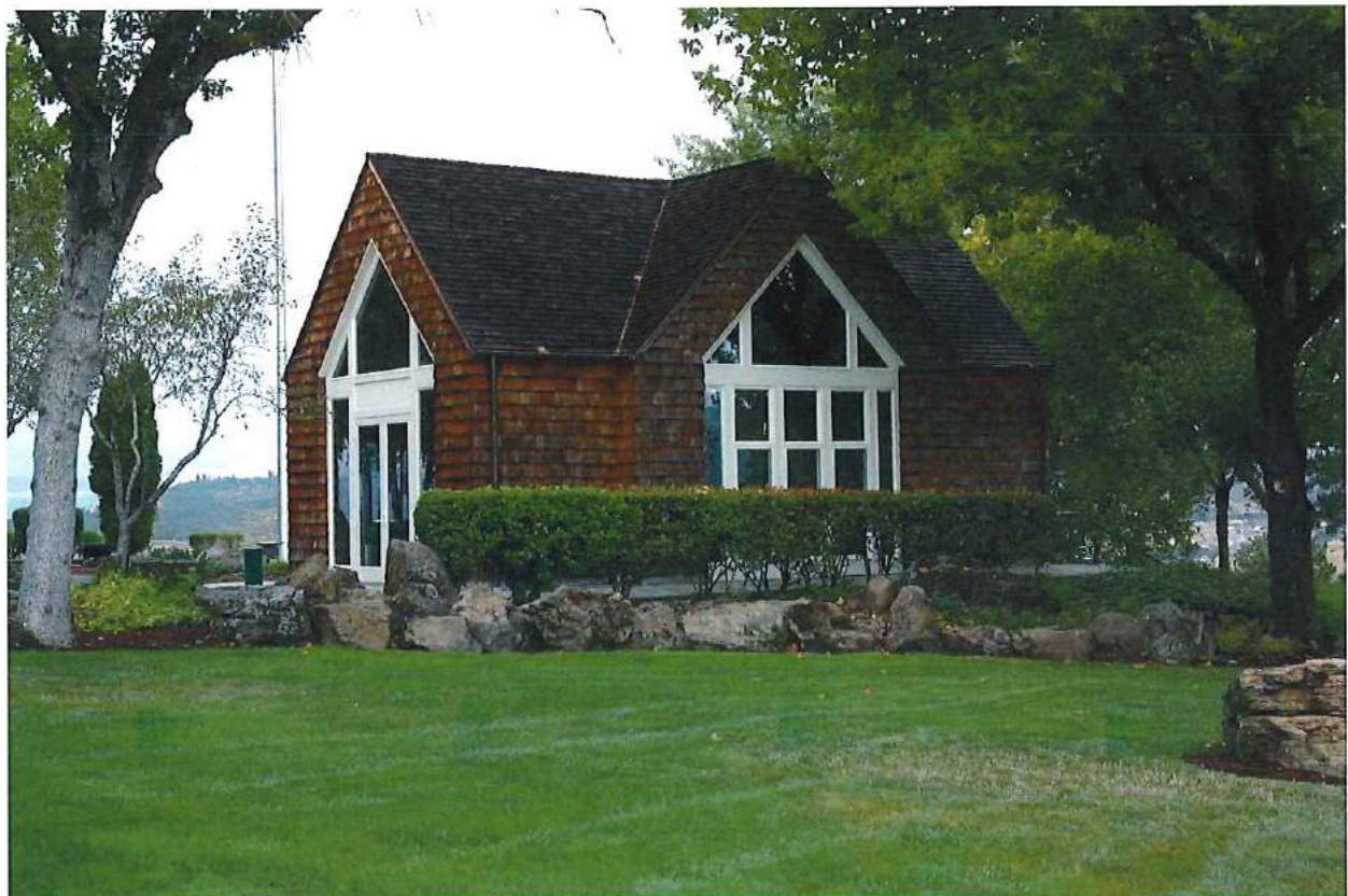
Photo 15 of 35: View to northwest, Committal shelter
