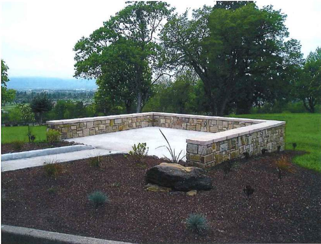
Photo 28 of 35: View to southwest, Rostrum
