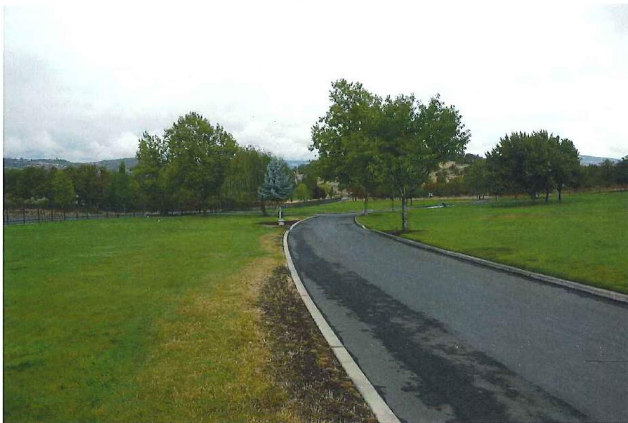
Photo 6 of 35: View to northwest, Section C and main entrance gate
