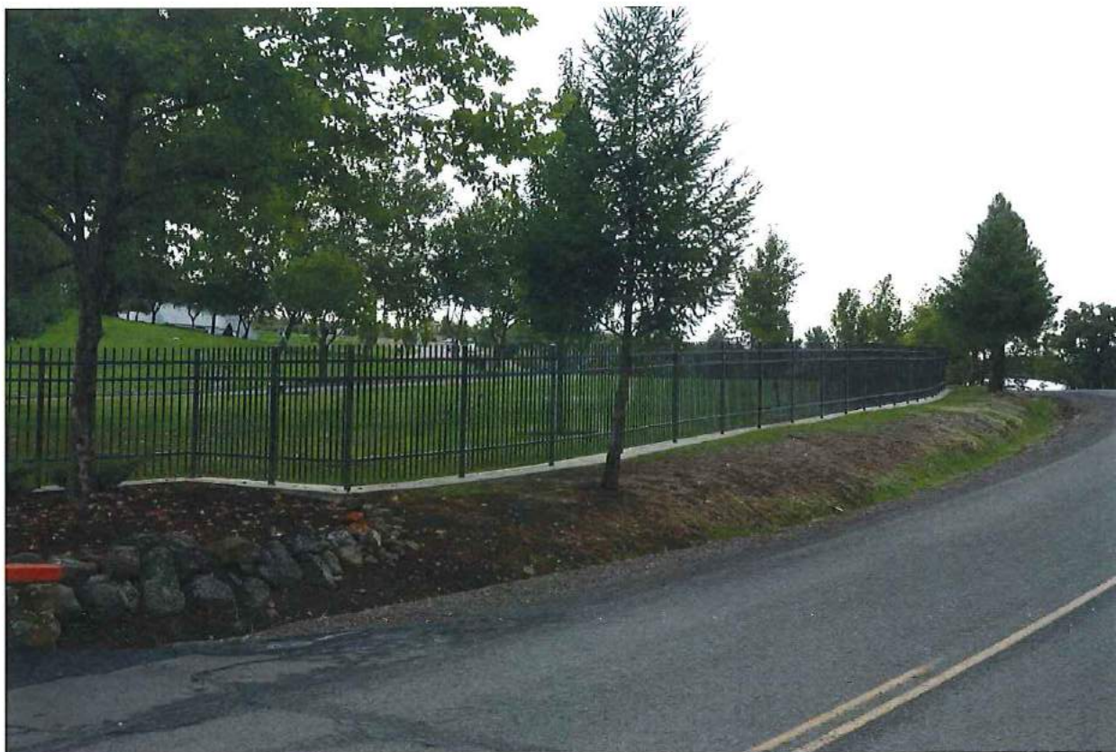
Photo 8 of 35: View to southeast, Perimeter fence
