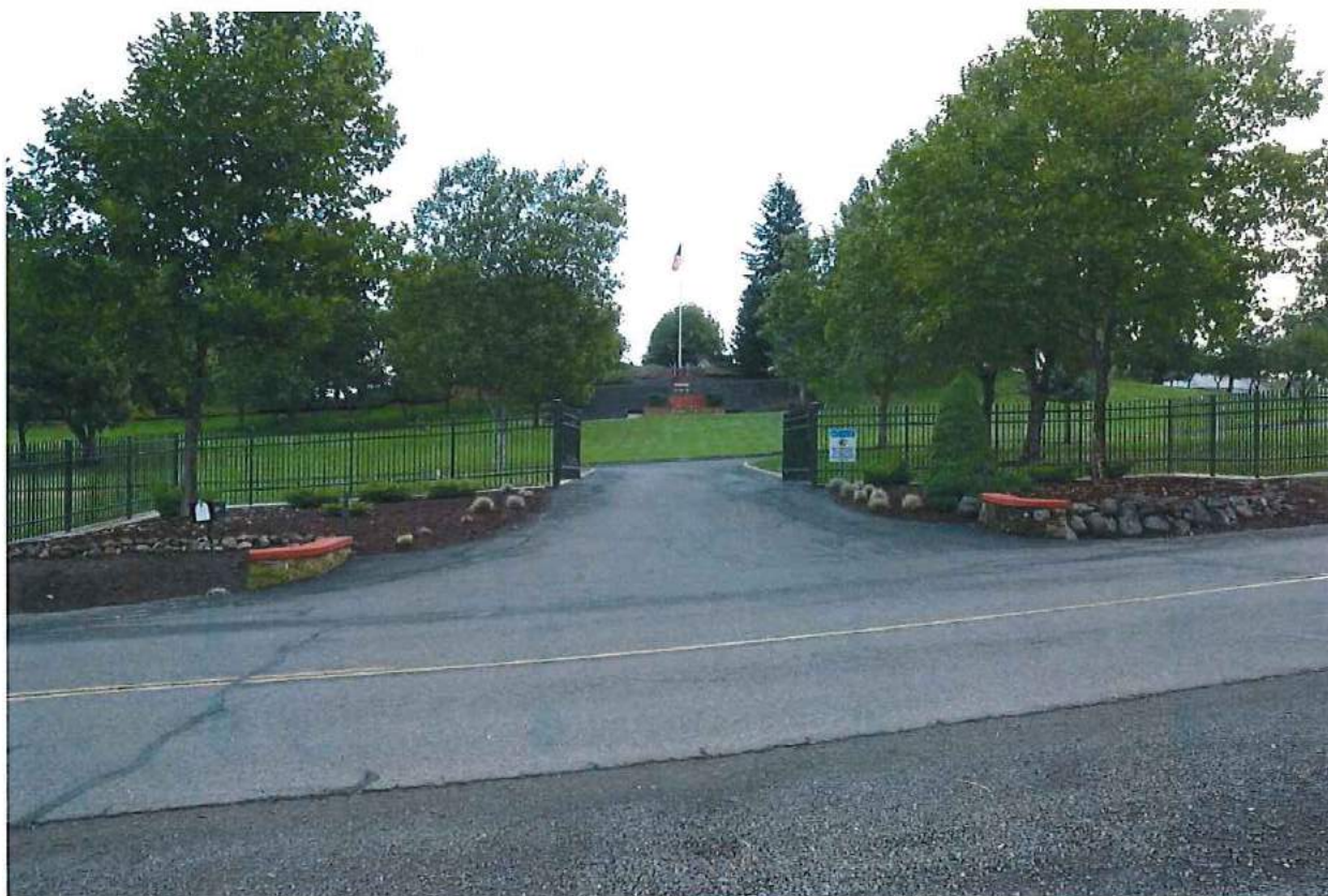
Photo 7 of 35: View to east, Main entrance gate
