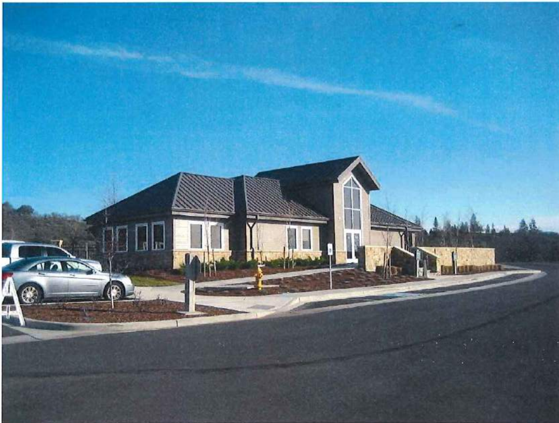
Photo 30 of 35: View to southeast, Administration Building
