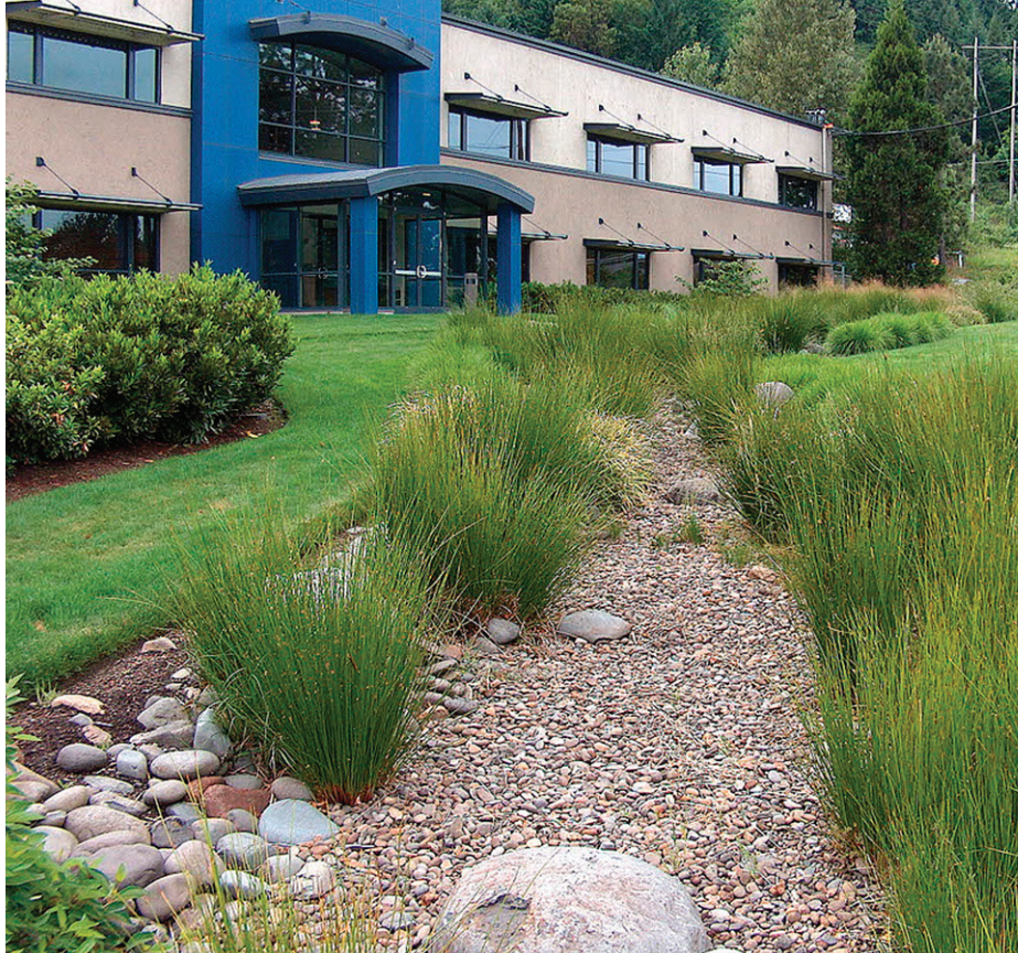
A dry bioswale in front of the Pepsi-Cola Bottling Co. building in Eugene where grasses, sedges, and rocks will capture and slow rainwater, allowing it to infiltrate into the ground below.
