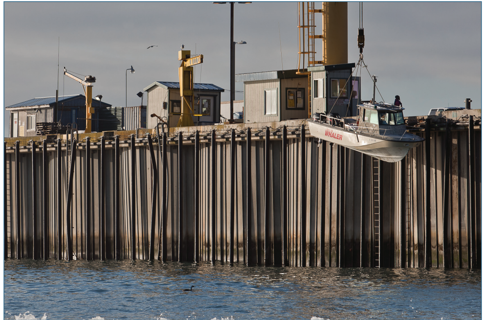
As the West Coast’s only dry dock, Port Orford launches fishing boats by crane (Photo: Heath Korvola).
