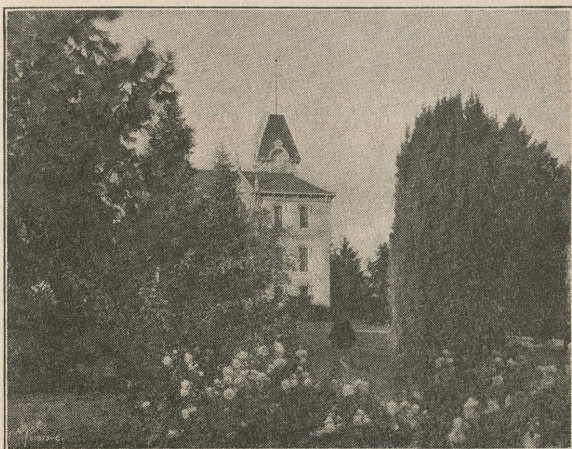
Administration Building, which contains the Workshop Theater, and the offices and studios of the School of Music
