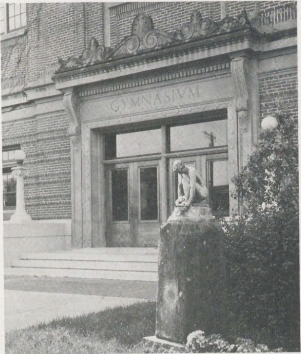
Main entrance to the Men's Gymnasium. Opposite the Memorial Union, this building is one of the main student centers of the Oregon State campus. Here convocations and student assemblies are called. Indoor athletic events are usually held in the great hall of the Gymnasium, which is the headquarters for Health and Physical Education and Intercollegiate Athletics.
