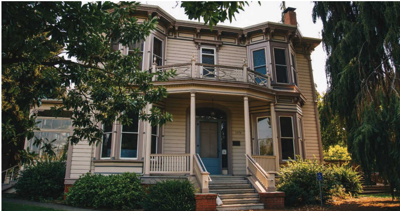
The Collier House has been at the same location since 1886; however, the university is planning to move the house in order to make space for a new classroom and faculty building. A timeline has yet to be set for the project. (Sarah Northrop)
