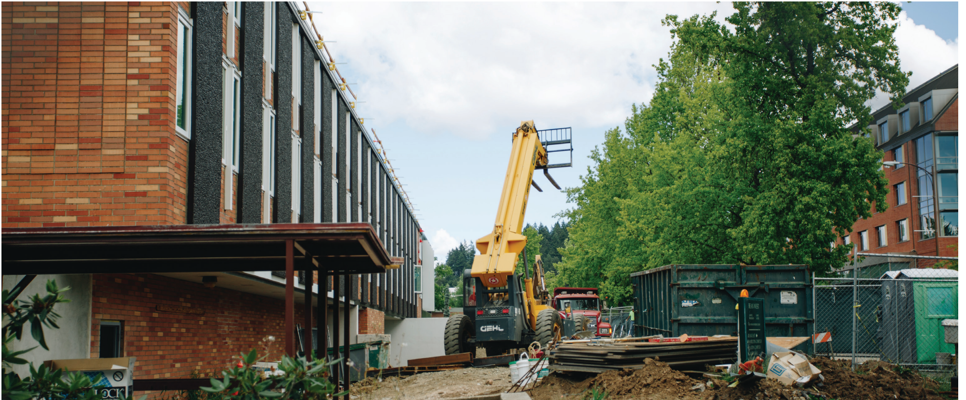
Bean Hall while under construction (Sarah Northrop/Emerald)
