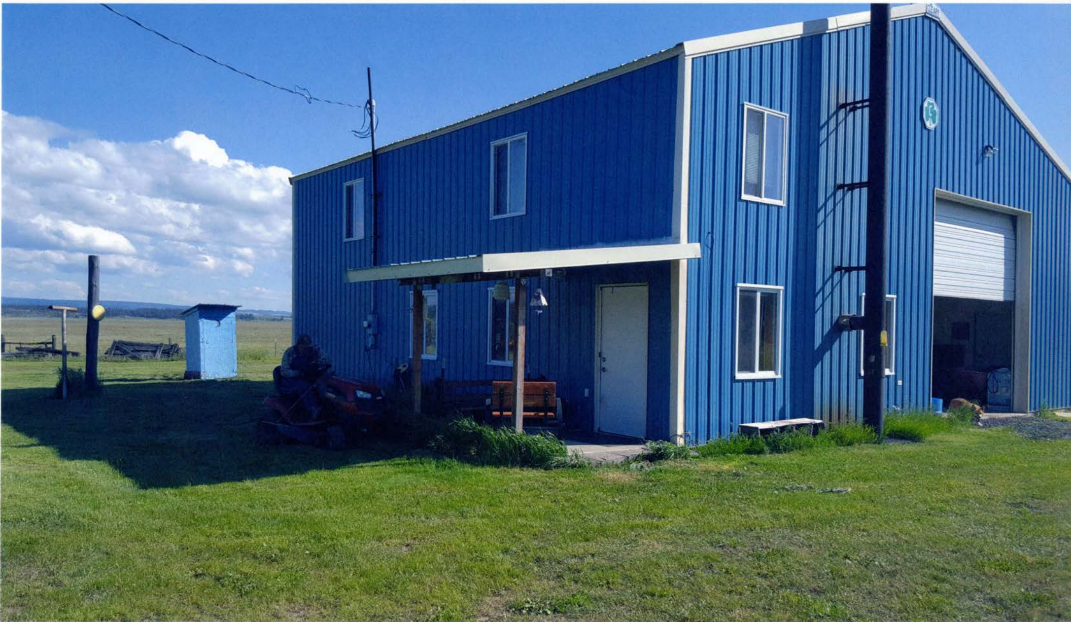
CURRENT HOUSE AND SHOP
