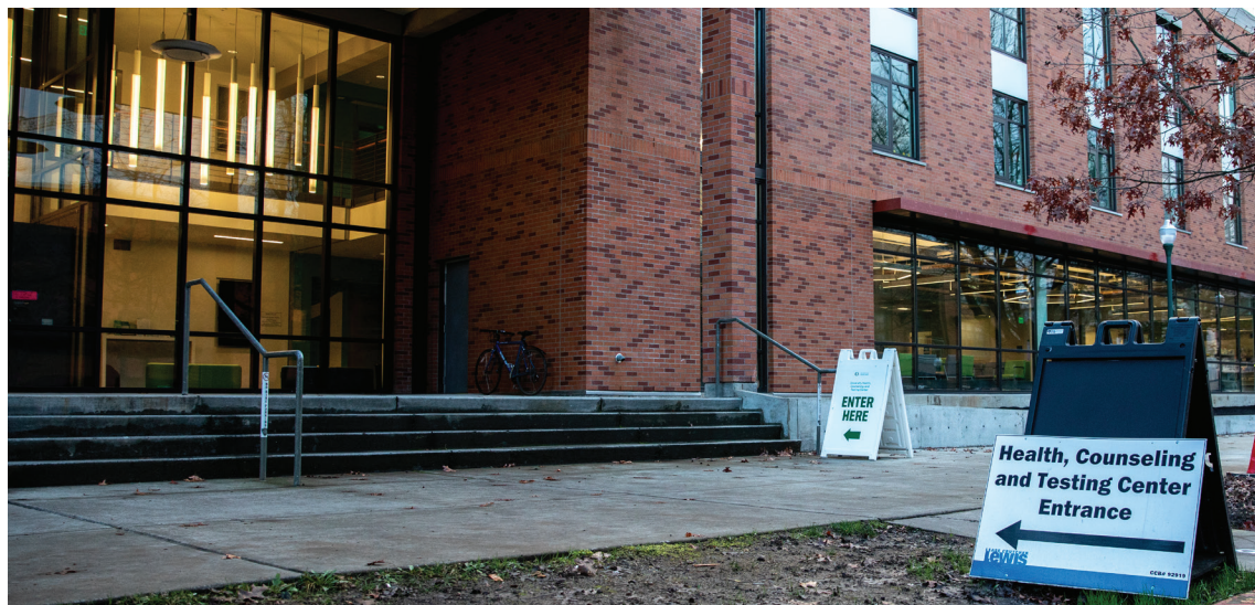
The University of Oregon Health Center undergoes construction on Jan. 17, 2020. (Maddie Knight/Emerald)
