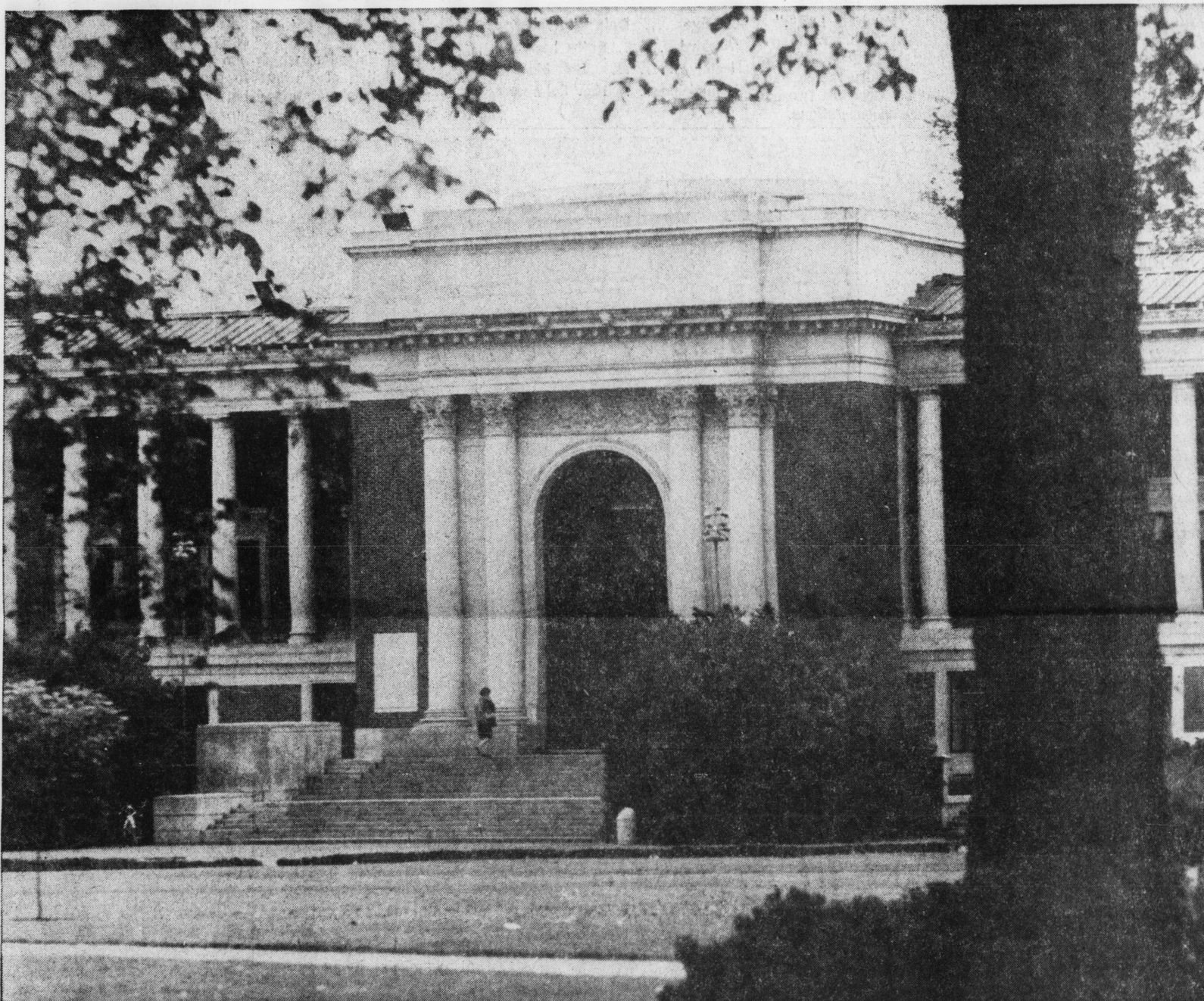
THE MEMORIAL UNION , the "living room of the campus," is the hub around which student activities revolve. The structure contains offices for student organizations and a student activity center. It has facilities for a snack bar and a cafeteria, music room, barbershop, book store, ballroom, billiard room, bowling lanes, art gallery, and meeting rooms of all types. The Memorial Union honors the memory of the men and women who have given their lives in the service of their country.
