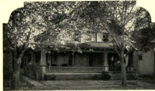
Eleventh and Jackson streets Installed 1930 Oregon State College
