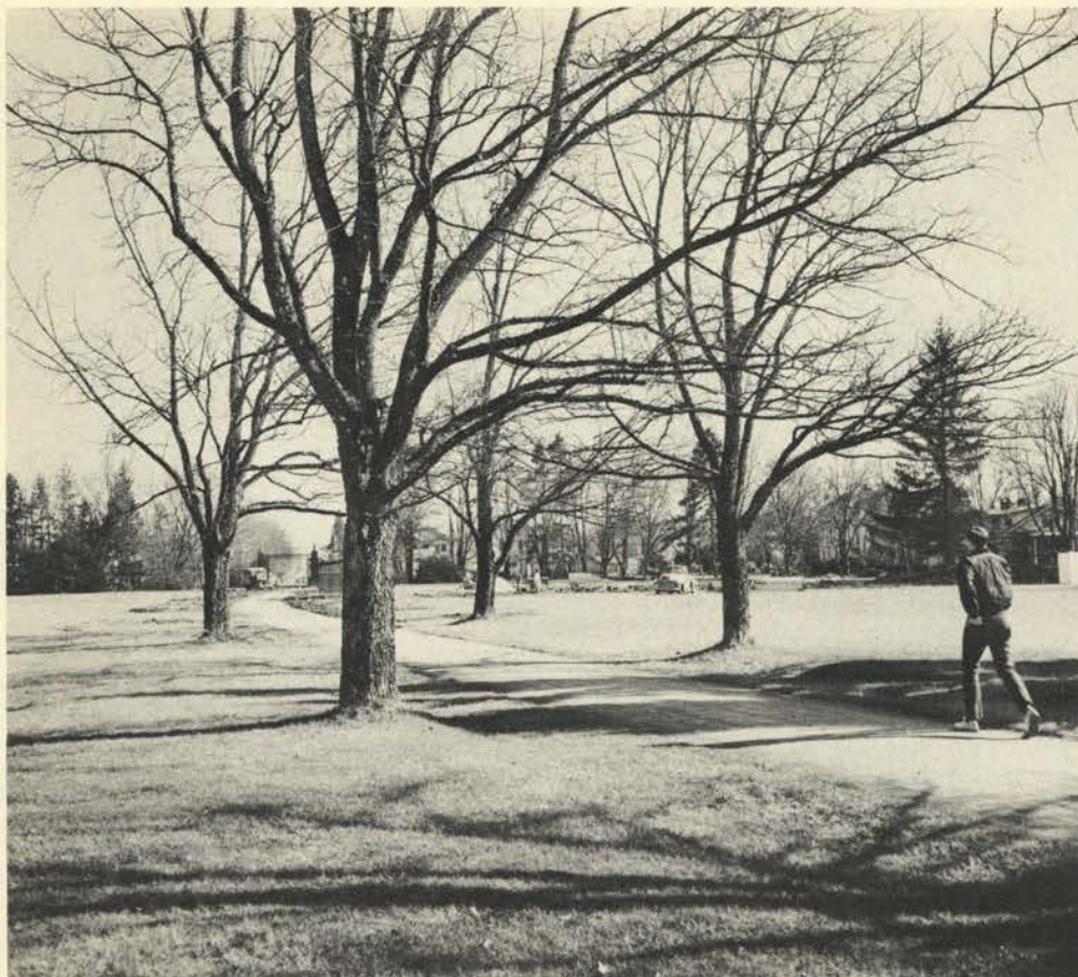
Lower Campus as it appeared before construction started on "operation facelift." In the background of the picture the lumber and materials are being moved into position. Many of the trees are already gone.
