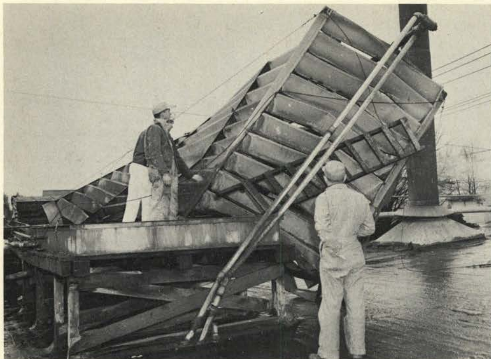
Corvallis city crews survey some of the damage caused by the twister, which brought a loss of about $100,000, as estimated by the city fire chief. The flooding Willamette River caused additional destruction.
