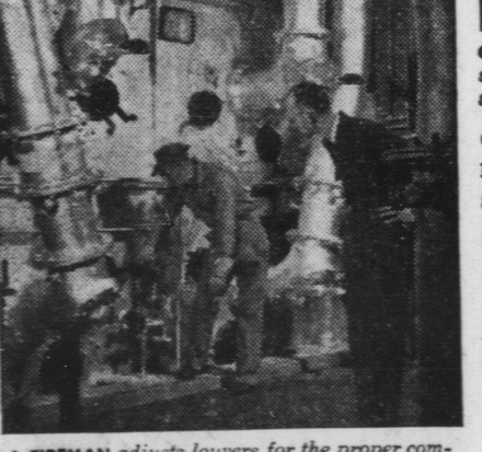
A FIREMAN adjusts lowers for the proper combustion of pulverized coal. Blown into furnace through pipes, it burns at 2500° F.
