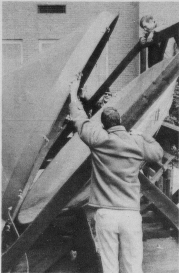
up onto the roof ourselves, but the easiest way would be to use a crane," he said.
